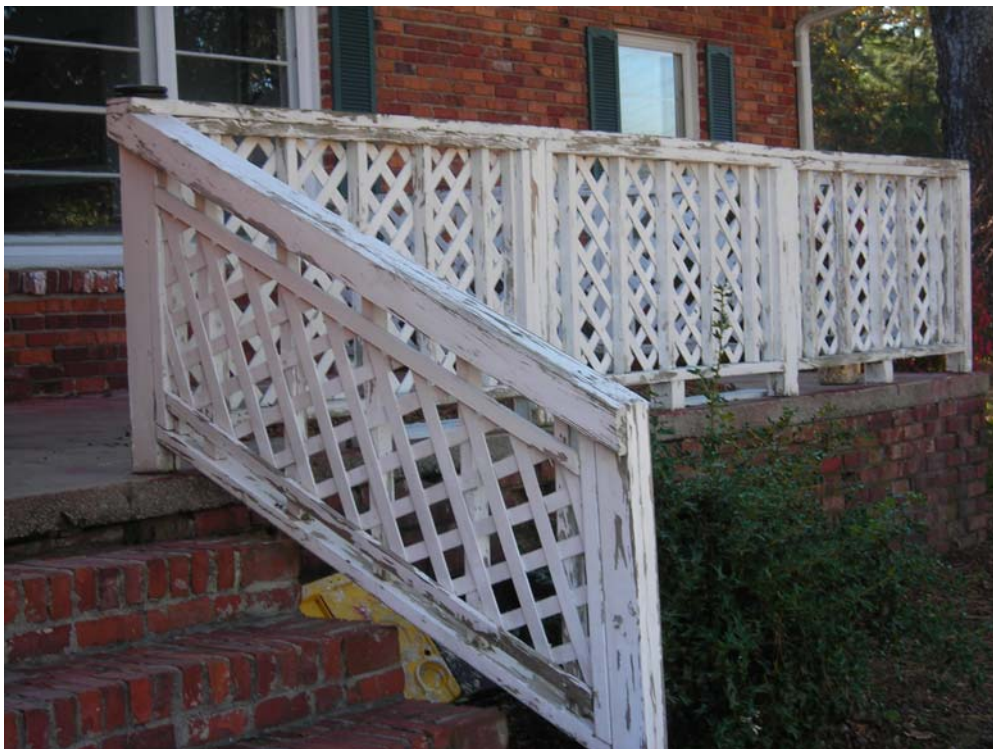
Picture 4 - Existing railing around porch and stairs
