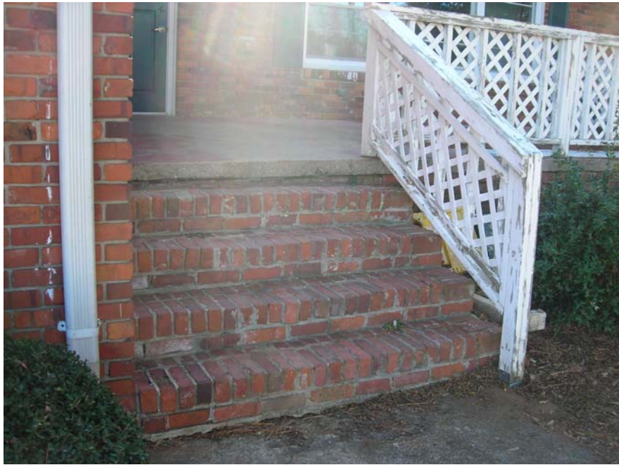
Picture 1 - Brick Steps leading from sidewalk to porch
